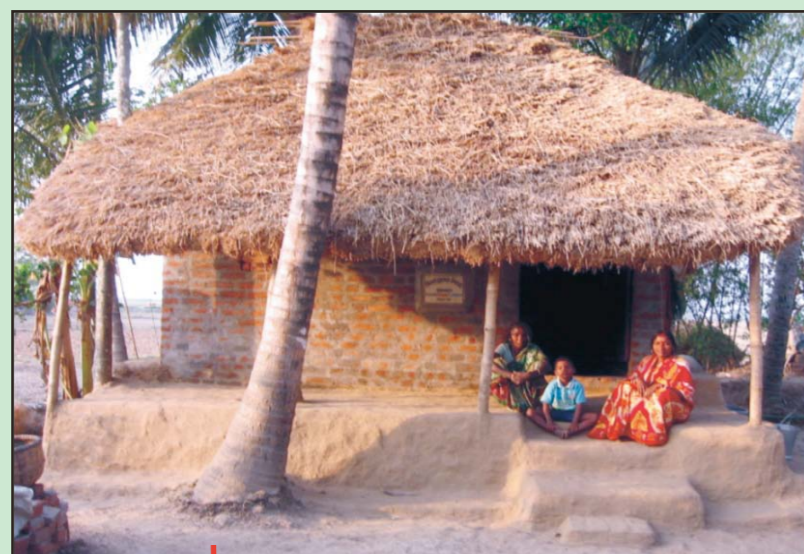
Newly constructed shelter on high raised plinth
