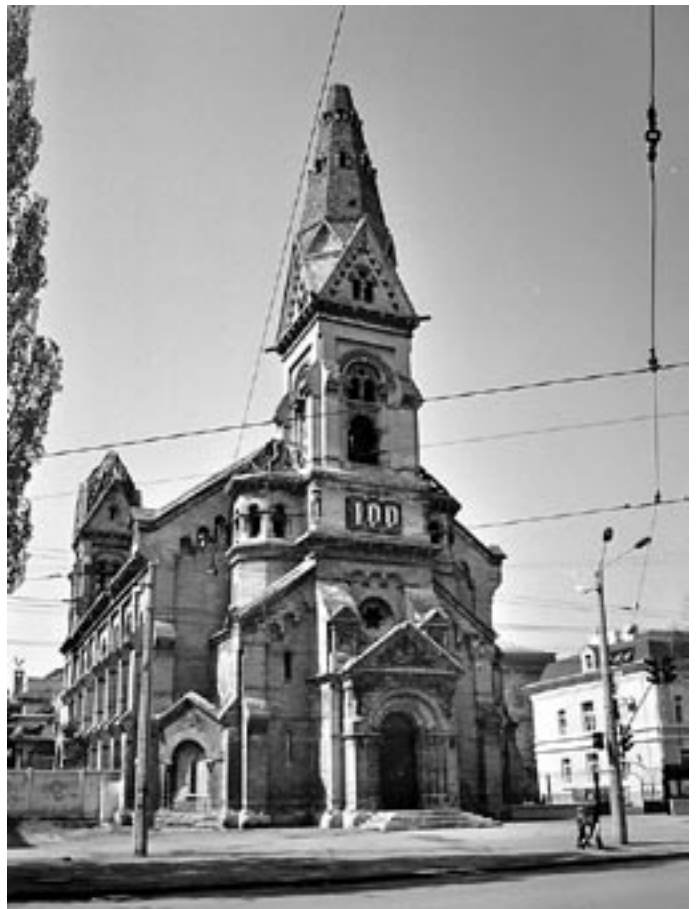
Reconstruction work has begun on St Paul's Church in Odessa, which was destroyed by fire in 1976. A new extension will include a "German Center" to accommodate agencies operating there for years. © LWF/D.-M. Grötzsch
