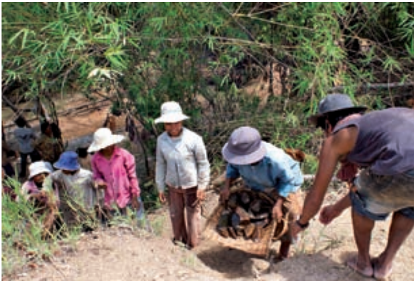
A chain of community bands at work, as Kraingskea Thbong villagers carry baskets of stones to fill in the water gate base. © LWF/DWS Cambodia/L. Ratna
