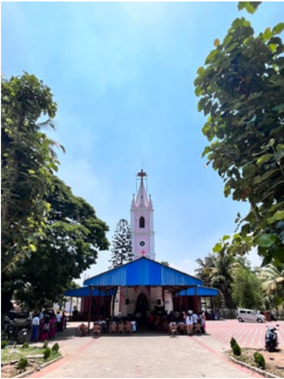
TELC Christ Church in Coimbatore, Tamil Nadu, India, was built in 1892. Photo: William Charles Jayaraj
